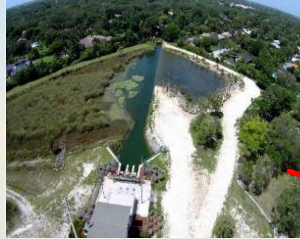
Deering Estate Pump Station (S-700)
