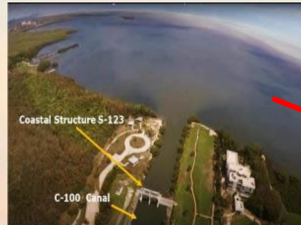
Coastal Structure S-123 on C-100 canal
